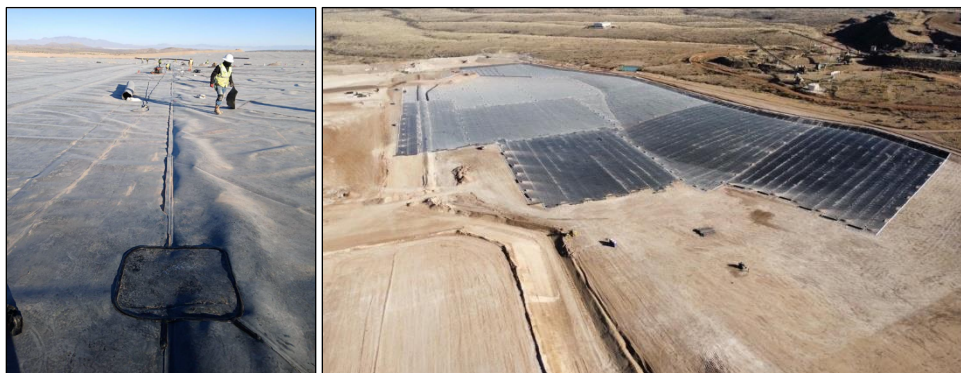
Figure 17-4: Liner Installation on Pad 5
