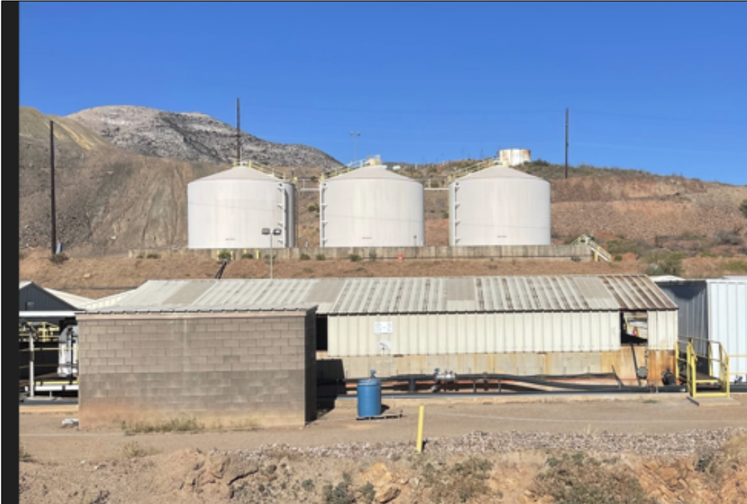
Figure 17-13: JCM Sulfuric Acid Tanks
